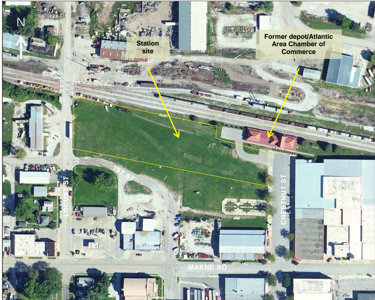
Figure 8.3-10: Atlantic Station Location
