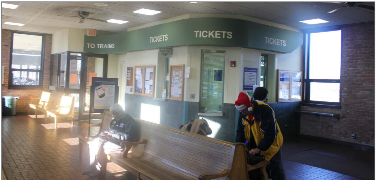
Figure 8.2-6: Interior View of Naperville Station Building
