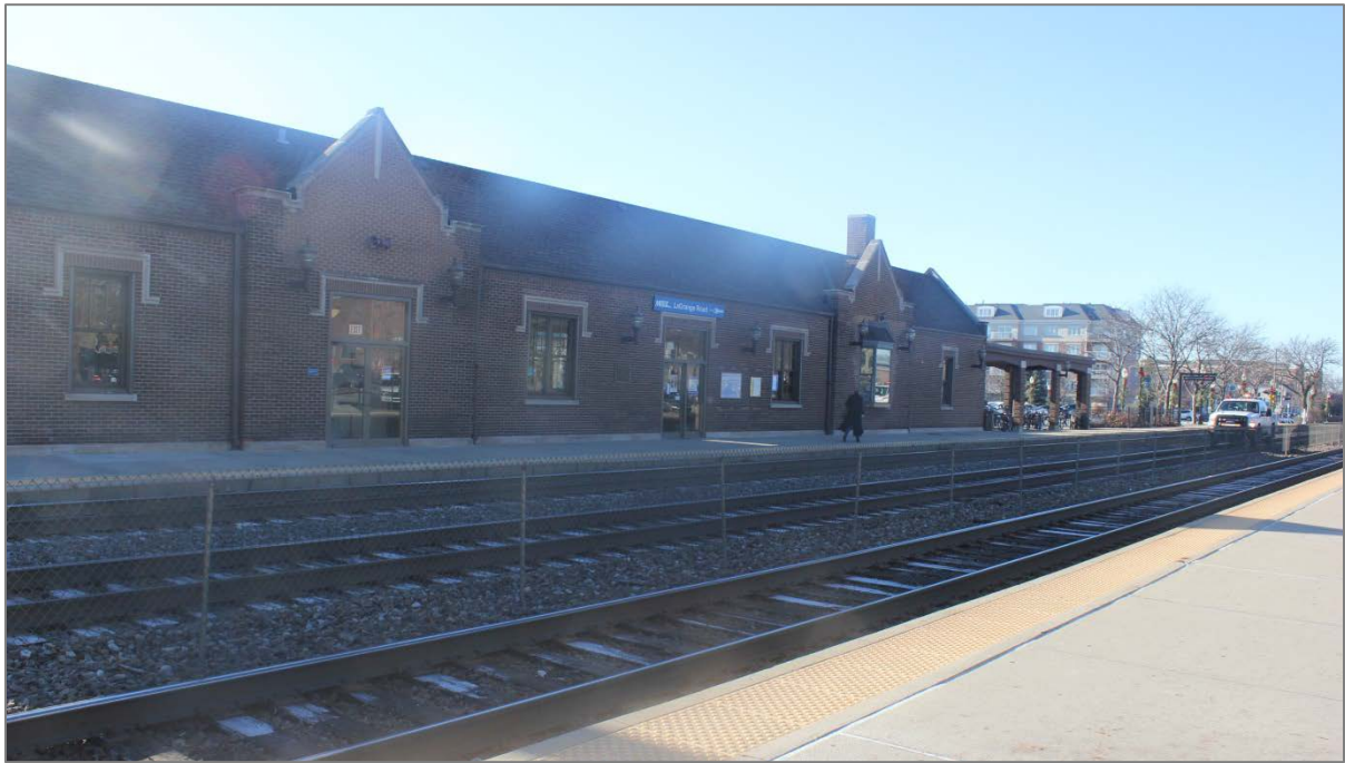
Figure 8.2-2: Exterior View of La Grange Road Station Building and Platforms
