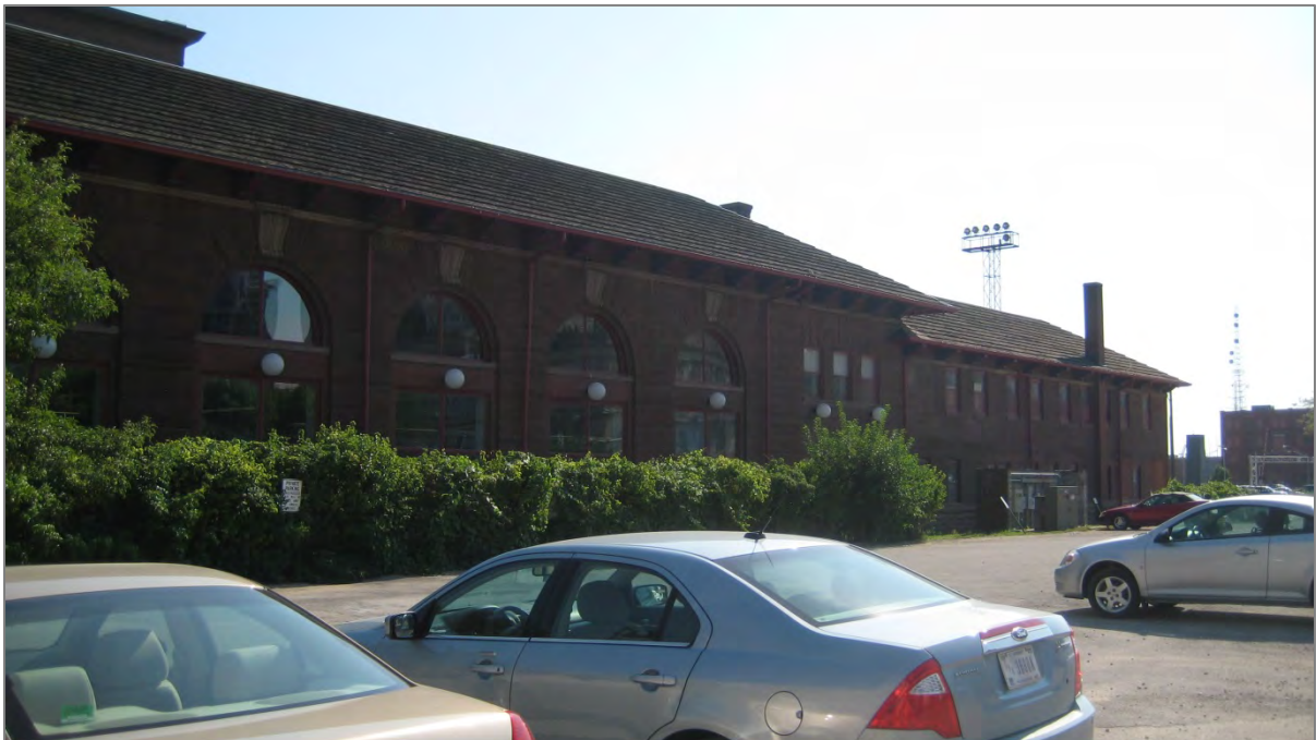
Figure 8.3-9: View of Station's North Side Looking from the Municipal Parking Lot
