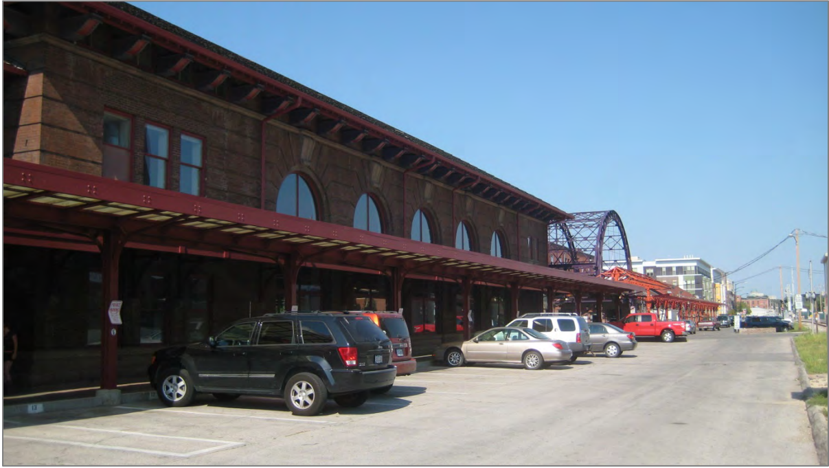
Figure 8.3-8: View of Station's South Side Adjacent to the Railroad Tracks
