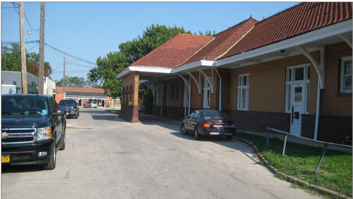
Figure 8.3-5: View of the Original Carriage Way on the North Side of the Depot along Wright Street
